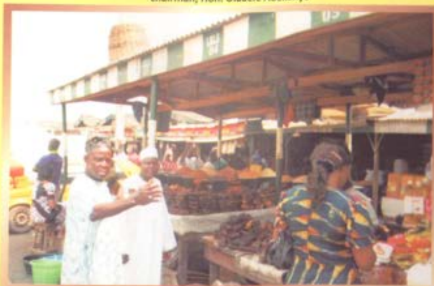
Part of 80 Units Completed Stalls by LMLG at White Sand Market under the Leadership of Hon. Oladele Adekanye Led Administration
