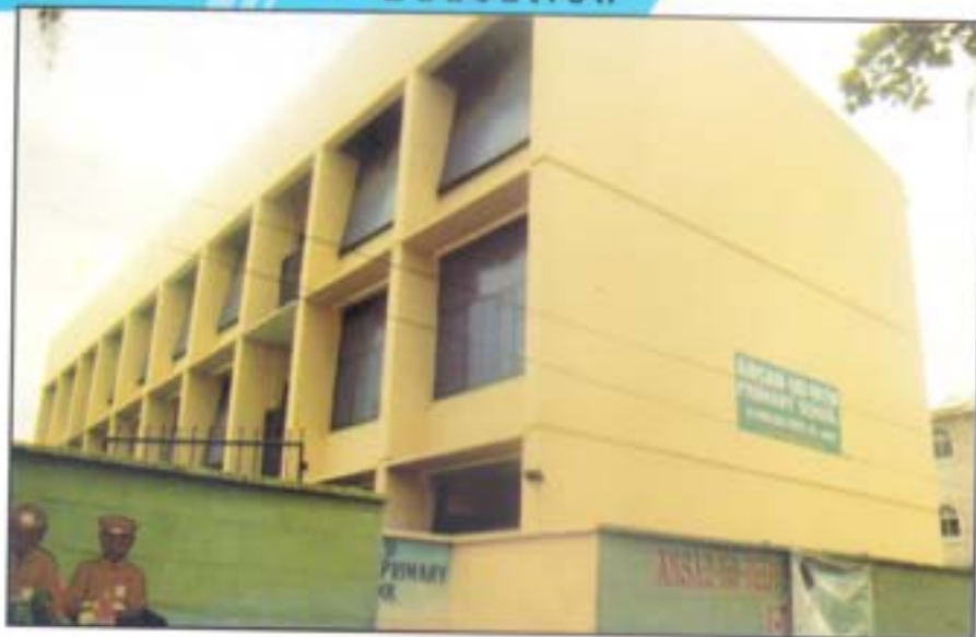
Replacement of roof, windows doors, repair of cracked walls and painting of AUD Primary School, Osholake
