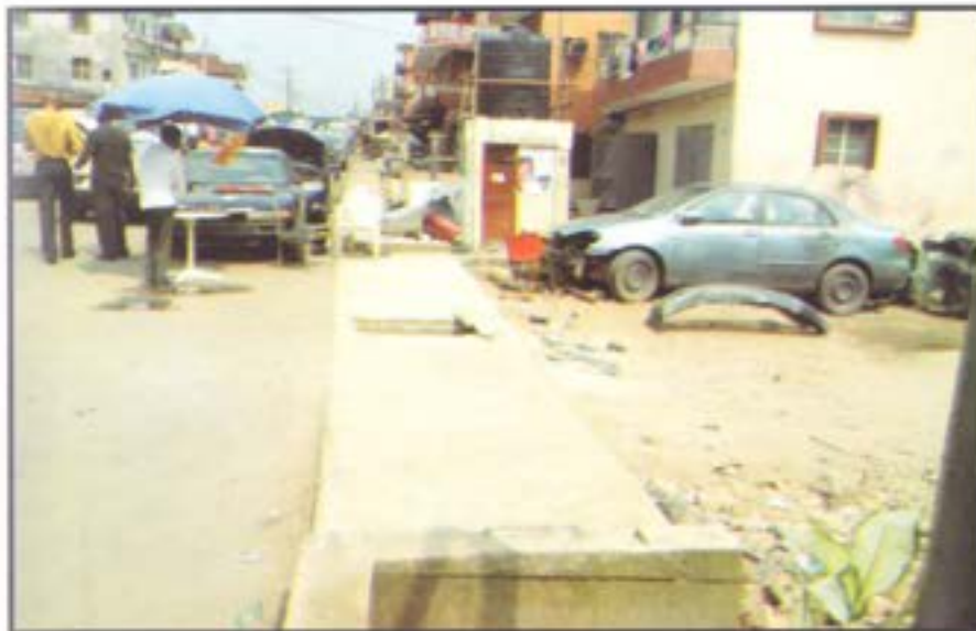
Completed reinforced concrete culvert along Lagos Street, by Osholake Street Ebute-Metta East
