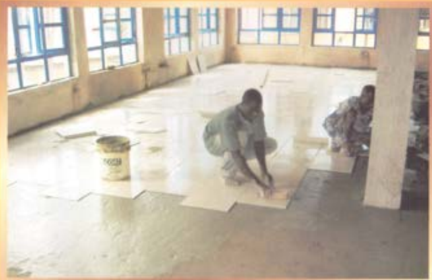
Floor tiling of the newly constructed secretariat in progress
