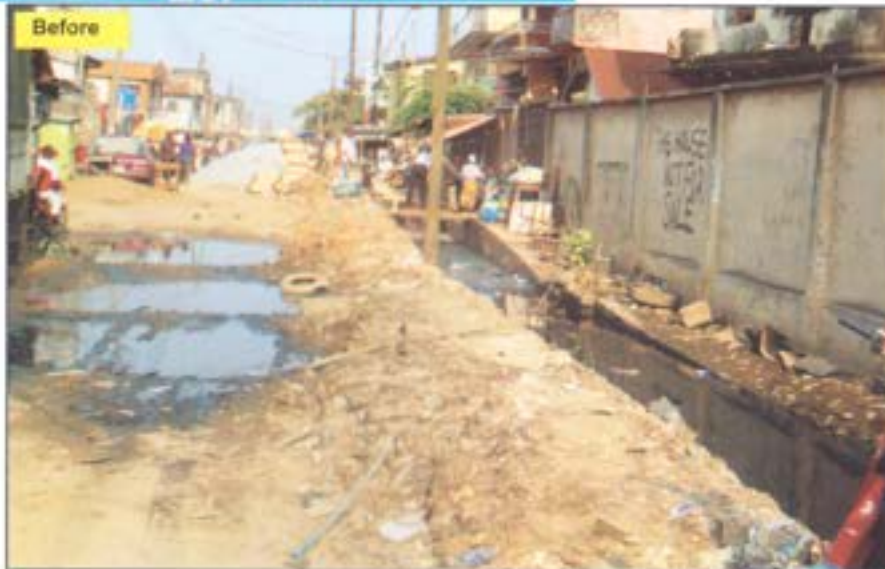
Lagos Street, Ebute-Metta East before construction
