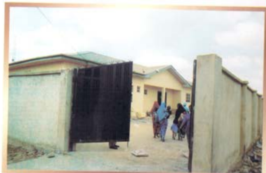
Completed perimeter fencing of otto PHC
