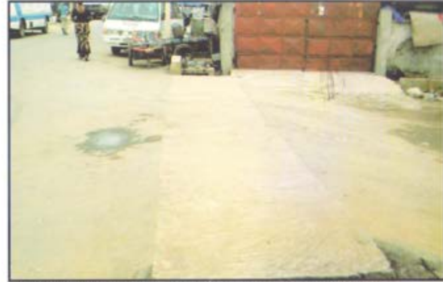
Completed reinforced concrete culvert along Lagos Street, by Odunfa, Ebute-Metta East
