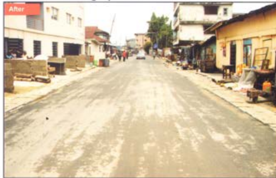
The 300m Ijero Road, Ebute-Metta West with double wall reinforced drainage system and concrete slab
