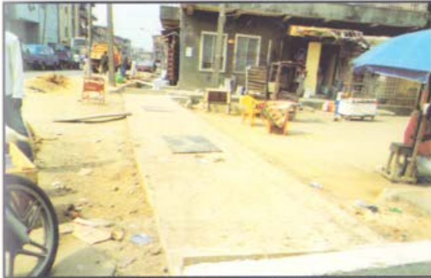
Completed reinforced concrete culvert along Lagos Street, by Borno Way, Ebute-Metta East
