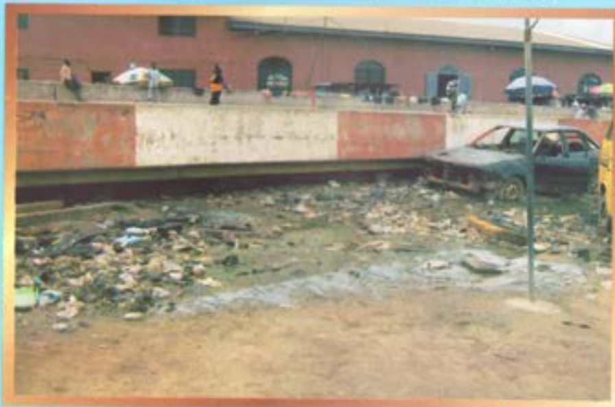
Okobaba football pitch surrounding wall before renovation
