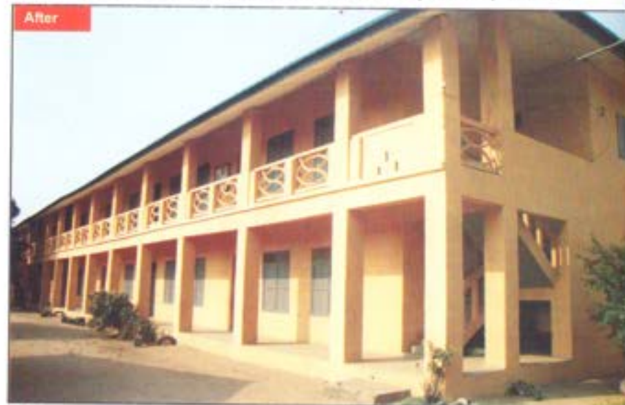
Replacement of roof, windows, doors, repair of cracked walls and painting of St Paul's Catholic Pry School, Costain
