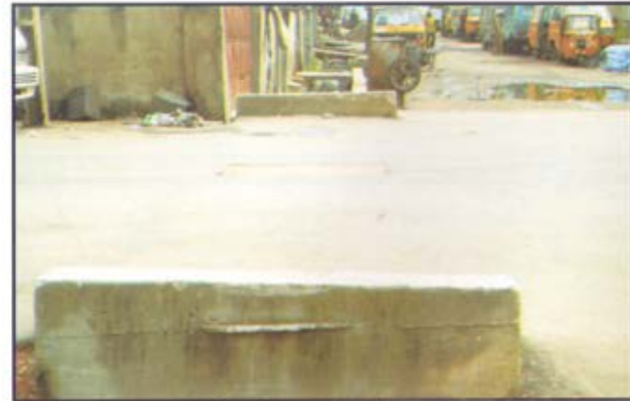
Completed reinforced concrete culvert on Lagos Street, Ebute-Metta East
