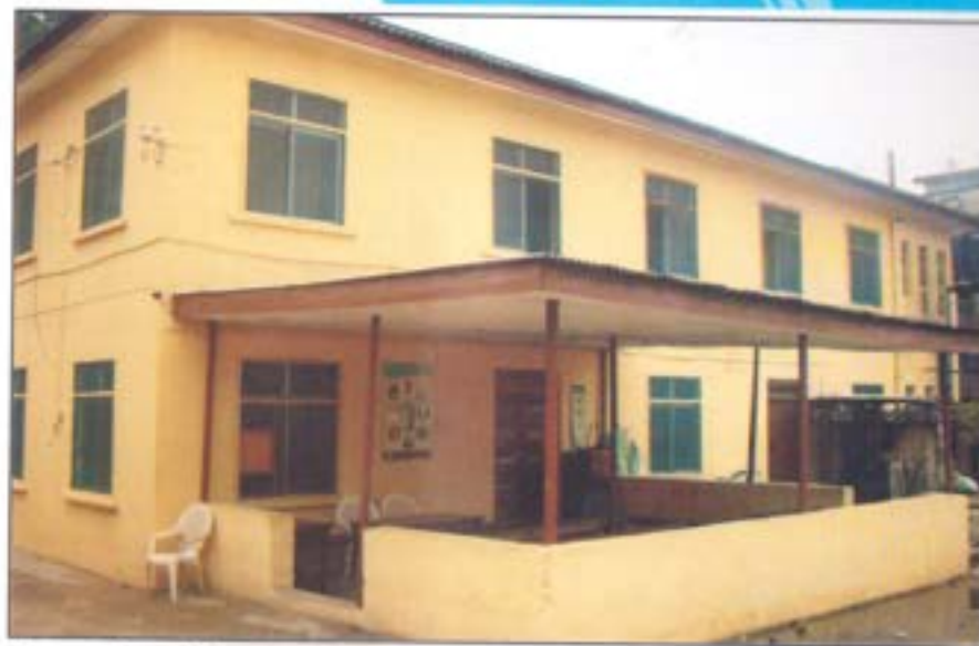
Rear view of the newly renovated Simpson Primary Health Centre
