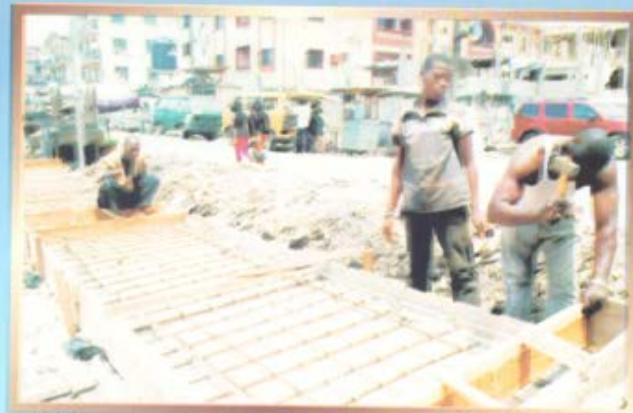
Reinforced concrete culvert on Odunfa Street, by Ondo Street, Ebute-Metta East during construction
