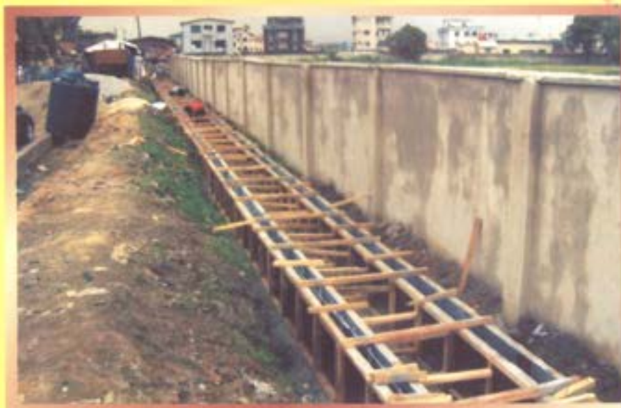
Drainage Construction work in progress on Moshalashi Street, Iponri
