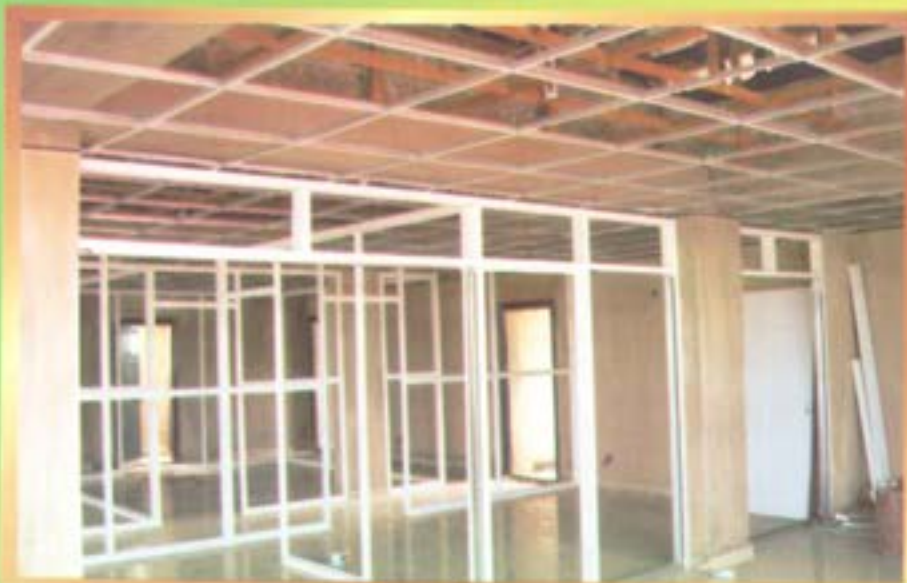
Aluminum partitioning of the newly constructed secretariat in progress
