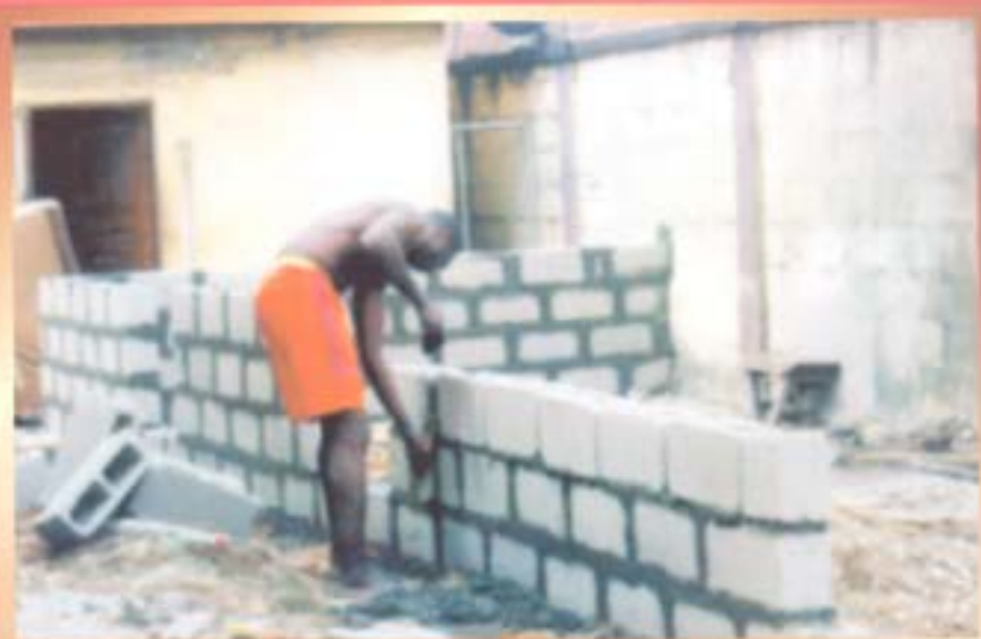
Construction of a new five-office building in progress
