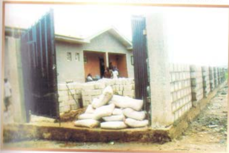
Perimeter fencing of Otto PHC in progress
