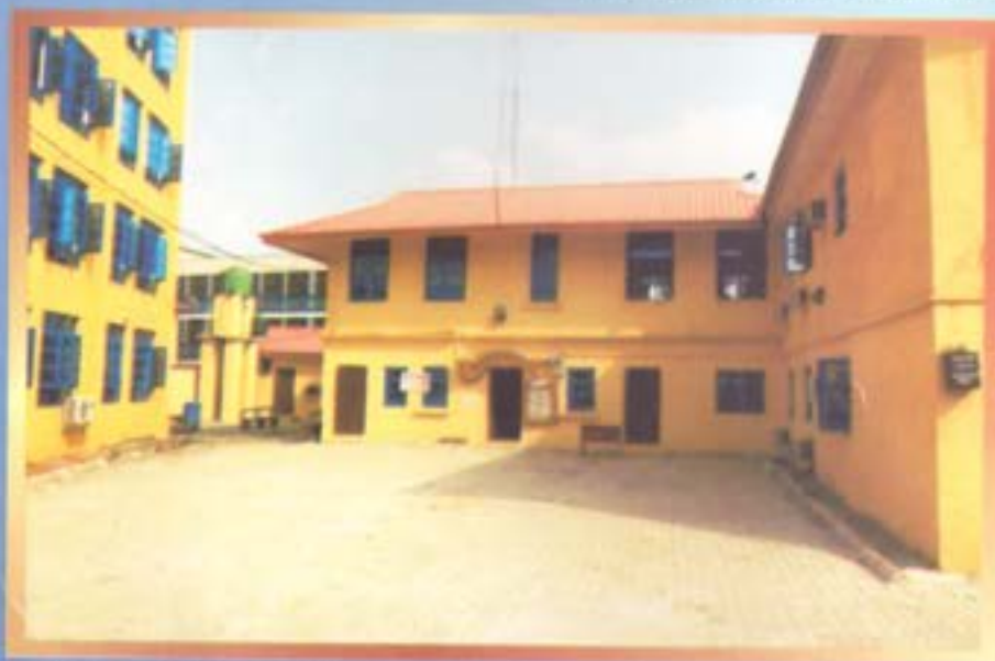
Setting of interlocking stones and general renovation completed
