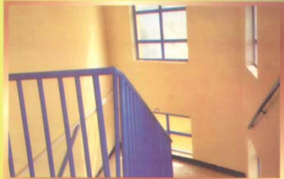
Completed wall POP with quality paint finishing
