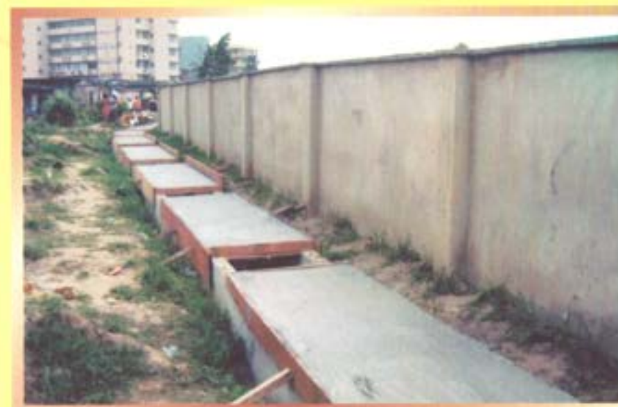
Completed reinforce concrete drainage system with concrete covered slab on Moshalashi Street Iponri
