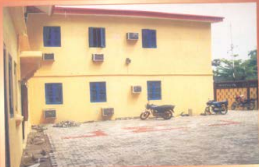
Old office block with interlocking stones after it was renovated
