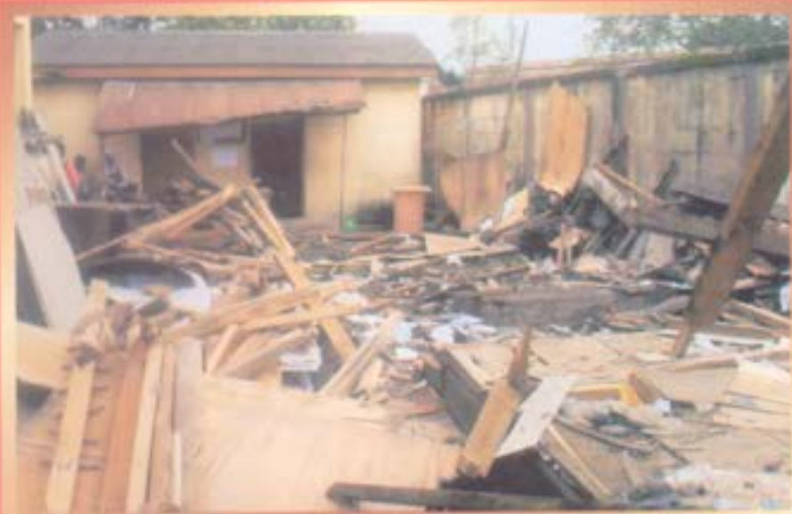
Demolition of old structures completed
