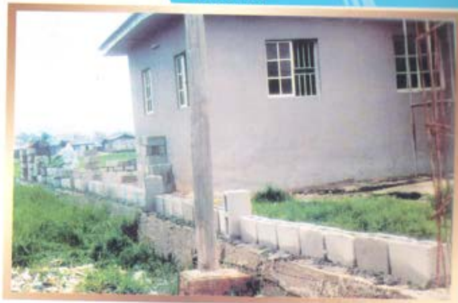
Perimeter fencing of Otto PHC in progress
