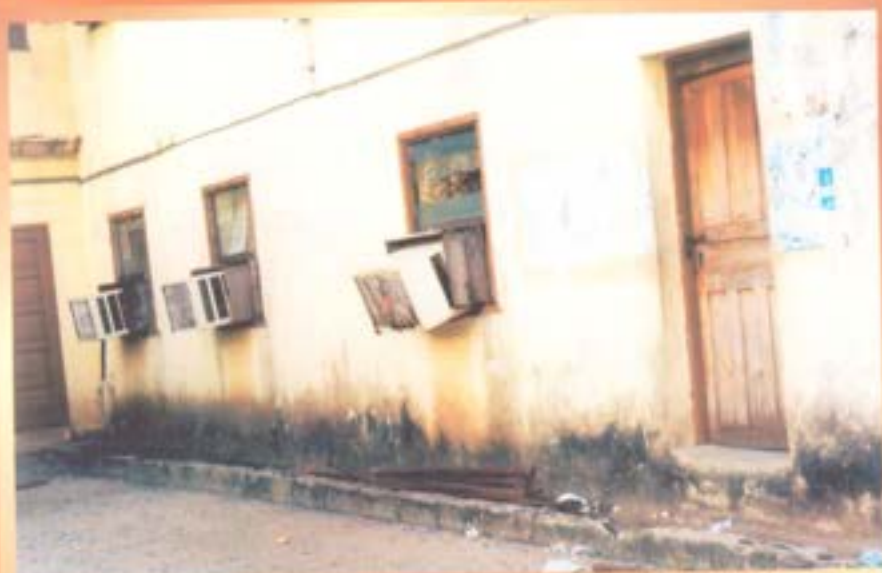
Old office block before renovation
