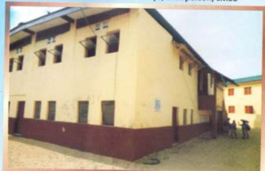
Newly renovated UNA Primary School, Odunfa
