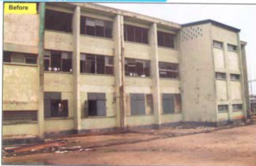
St Peter's Catholic Primary School, Costain before renovation
