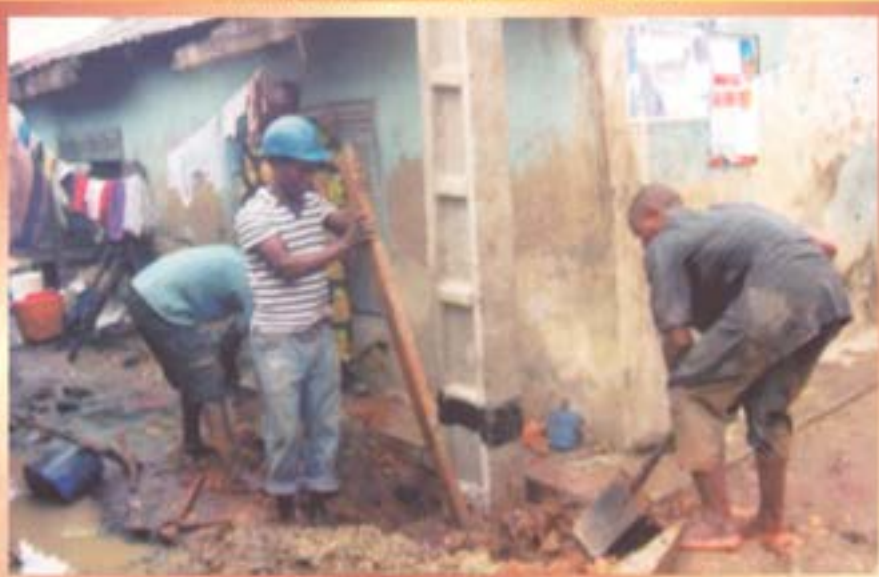
Erection of New Electric Poles on Mosalashi Street, Iponri preparatory to Road Construction
