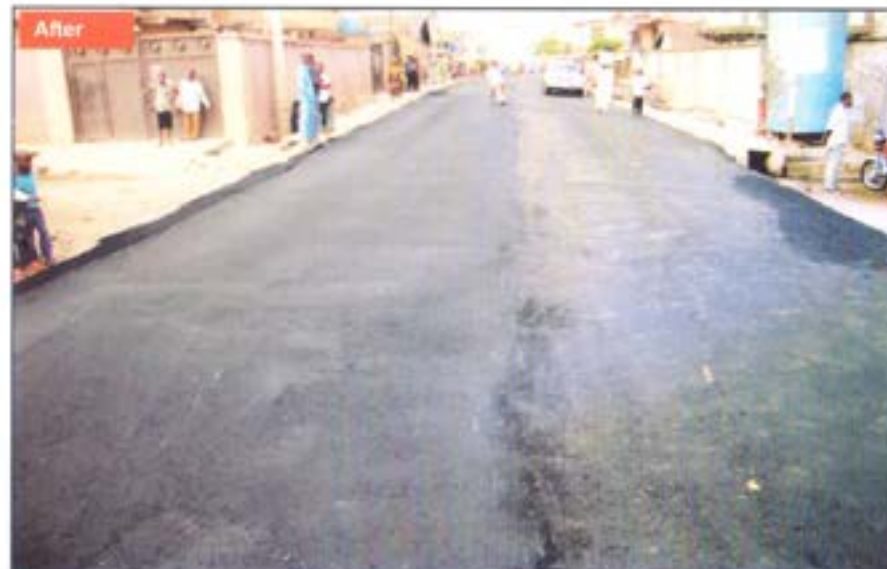
Completed 430m long Lagos Street, Ebute-Metta East with double wall reinforced drainage system and concrete slab
