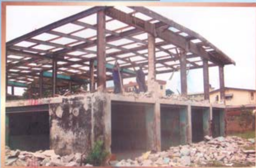
Demolition of structurally defective Ansar-Ud-Deen (AUD) Public School, Odunfa
