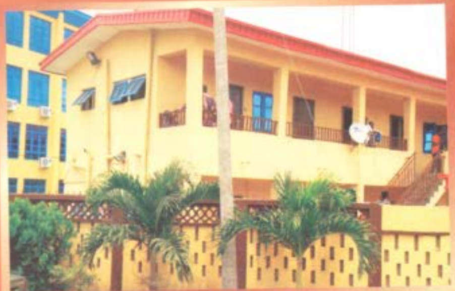
Council secretariat building after renovation
