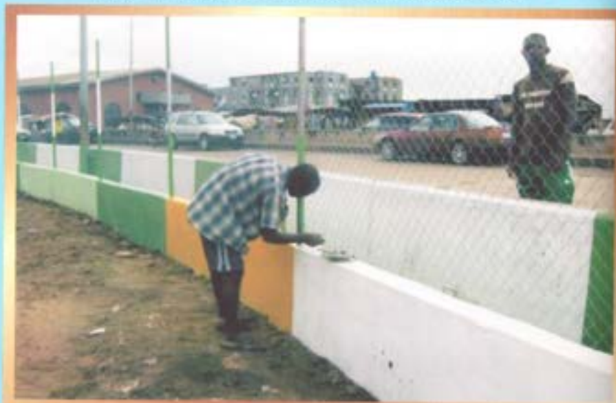
Completed Okobaba football pitch surrounding wall with barbed wire after renovation
