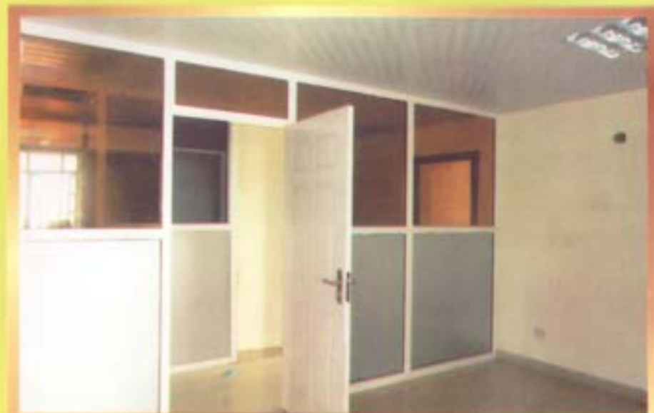
Completed aluminum partitioning
