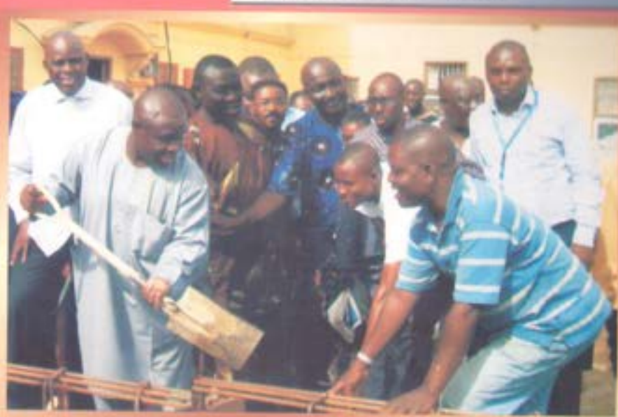
Hon. Adekanye laying the foundation of the council secretariat
