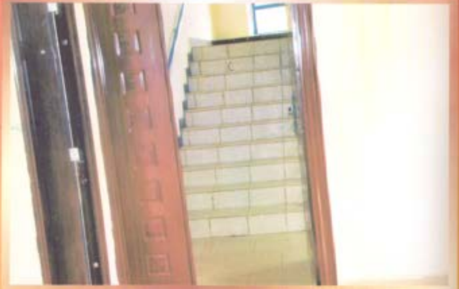
Part of the interior completed with tiles and quality paints
