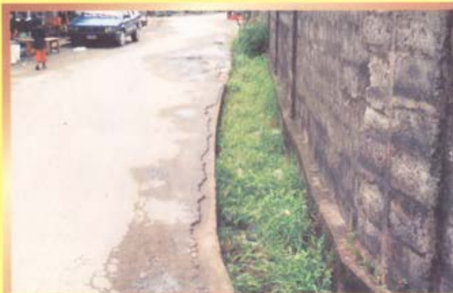
Drainage on Moshalashi Street, Iponri before construction
