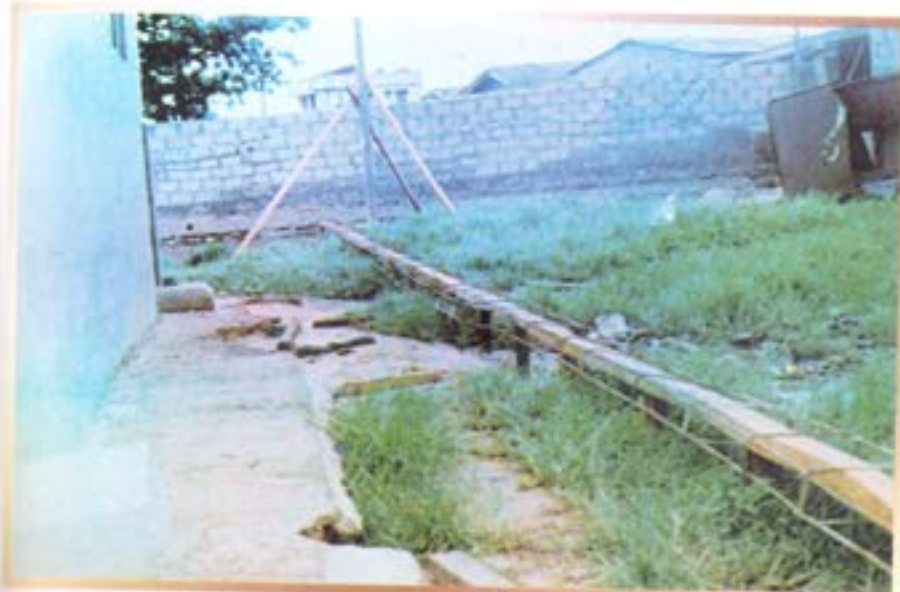
Frame work of the raft foundation for the perimeter fencing of Otto PHC
