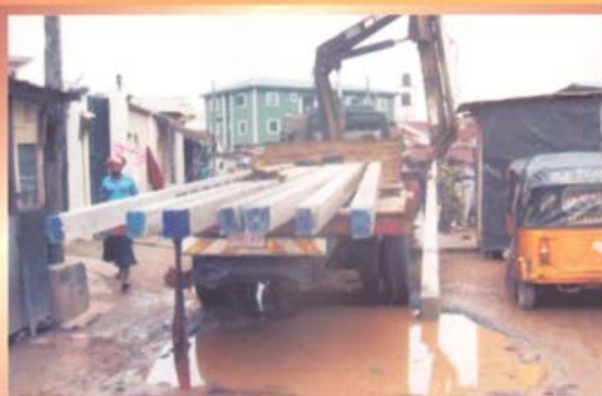
Some of the new electric poles meant for erection on Mosalashi Street, Iponri, preparatory to road construction
