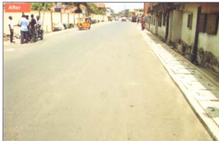
The 600m road with double wall reinforced drainage system and concrete slab
