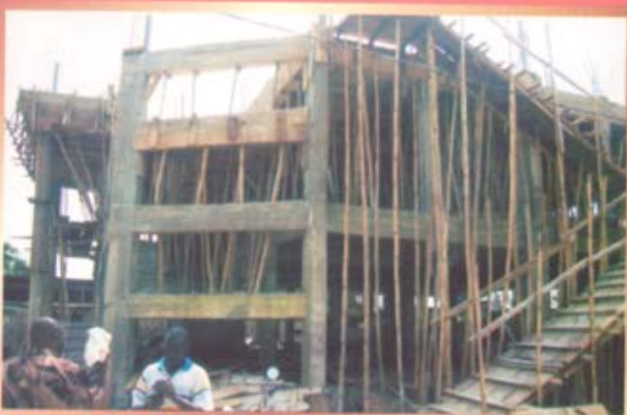
Ongoing construction of the new council secretariat building
