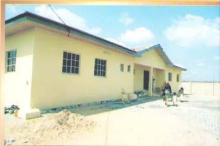
The PHC premises with interlocking stone laying in progress
