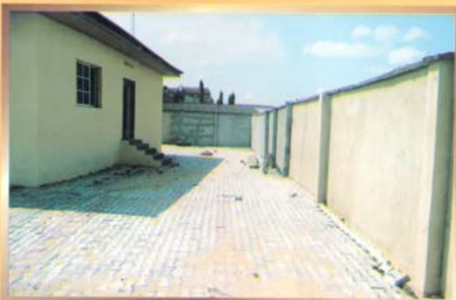
Rear view of the PHC completely fenced with interlocking stones
