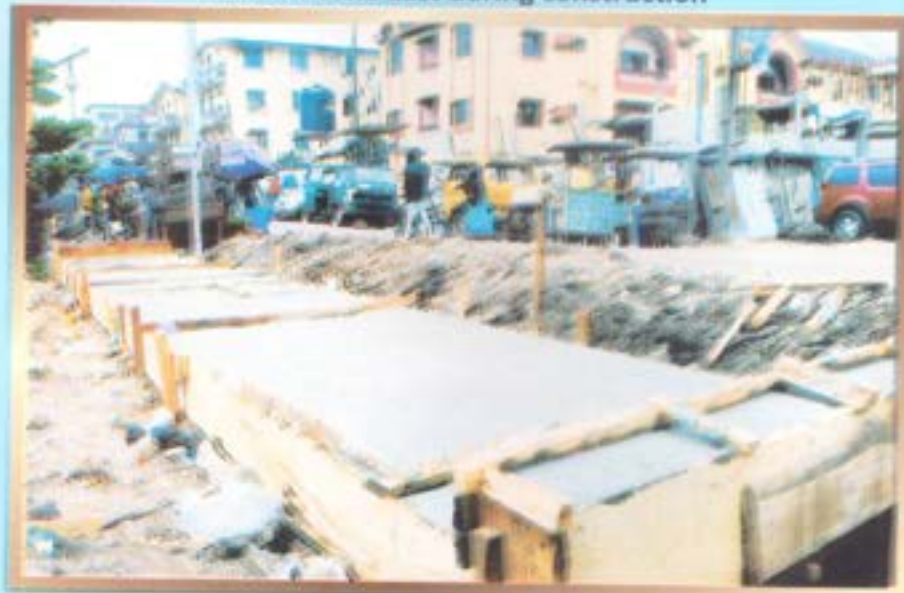
Reinforced concrete culvert on Odunfa Street, by Ondo Street, Ebute-Metta East during construction
