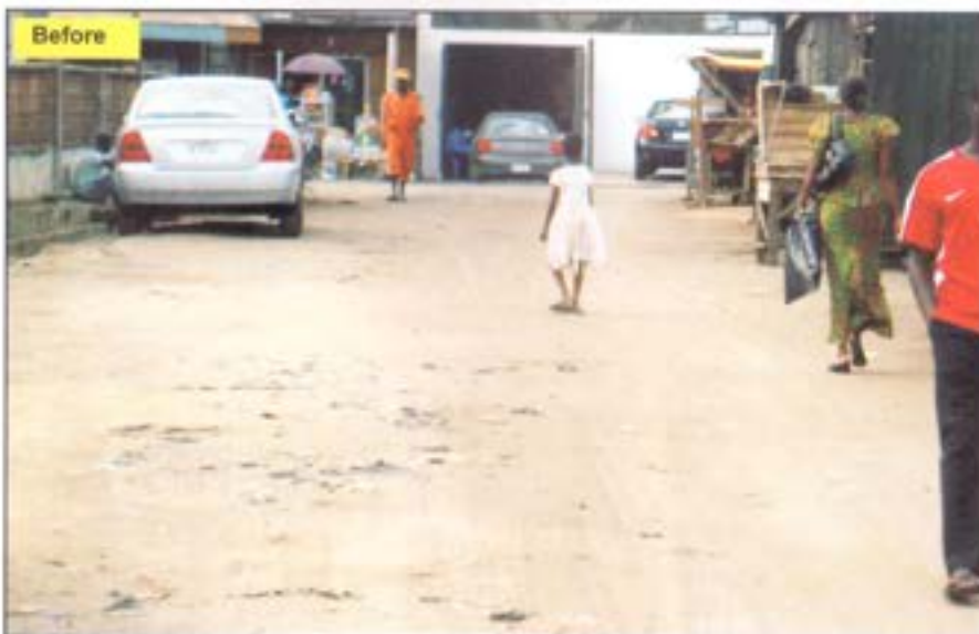
New Town Road, Ebute Metta West before construction
