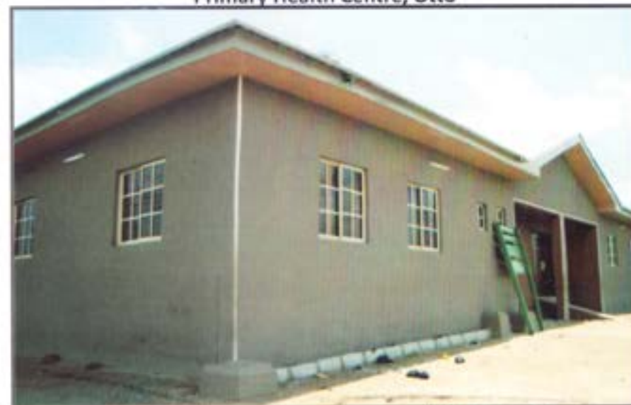
Completed ultra-modern Primary Health Centre, Otto
