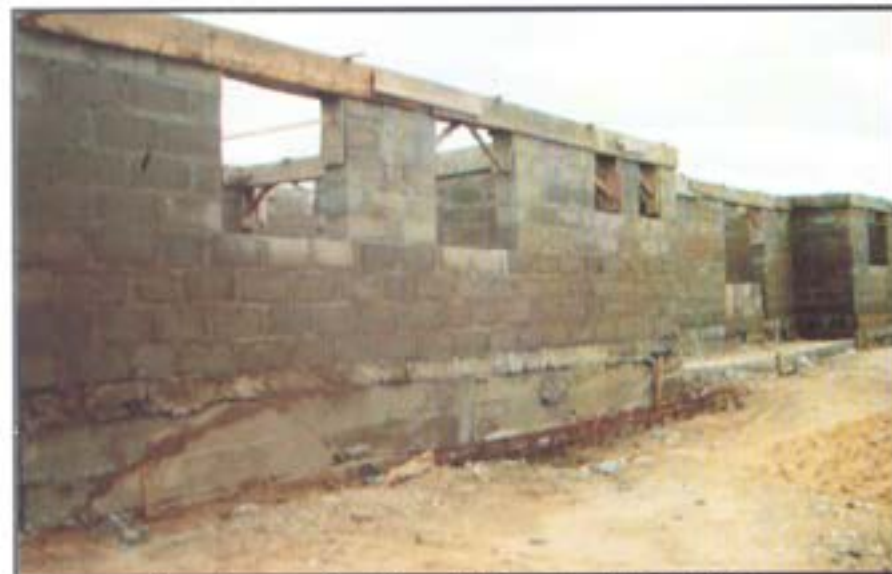
Ongoing construction of the new ultra-modern Primary Health Centre, Otto
