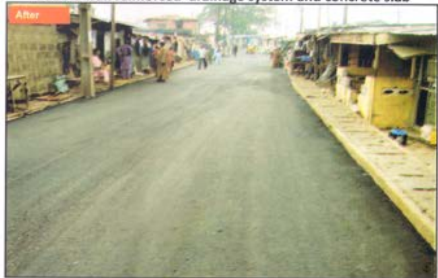
Completed 685m long Oba Ganiyu Odesanya Road with double wall reinforced drainage system and concrete slab
