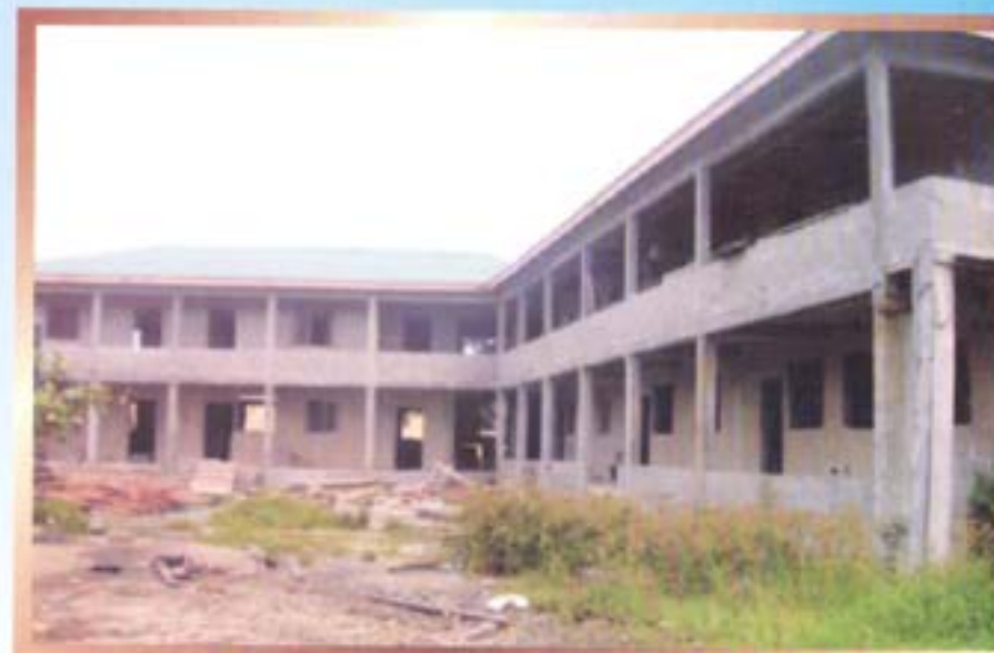
Construction of a new AUD Public Primary School in progress with 12 classroom, 4 toilets and 4 offices
