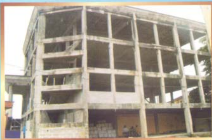
Construction work in progress (Side view)
