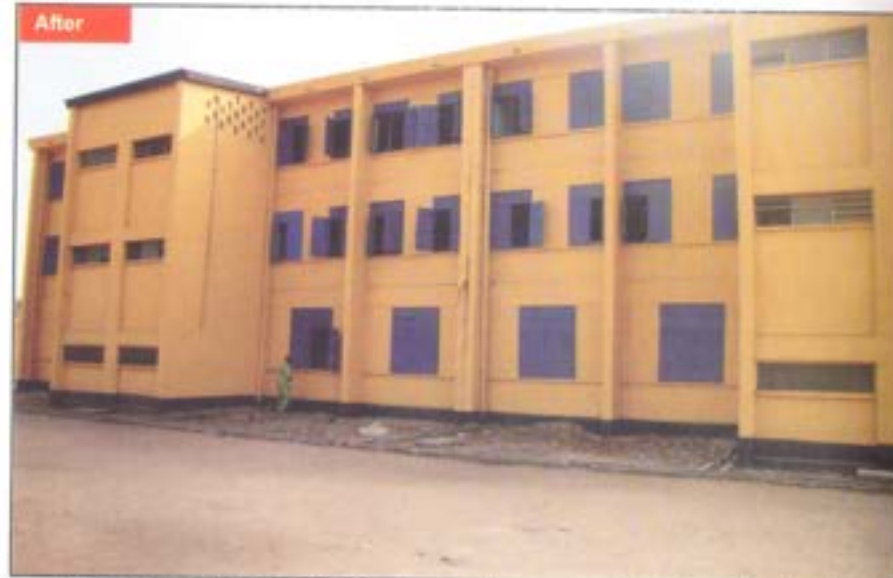
Replacement of roof, windows, doors, repair of cracked walls and painting of St Peter's Catholic Pry School, Costain
