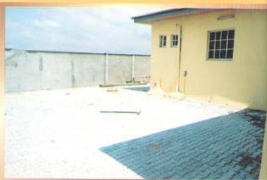
The ultra-modern PHC fully completed with interlocking stones and fence
