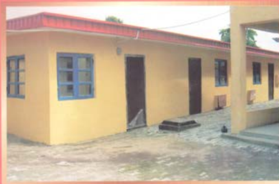
Completed five office rooms
