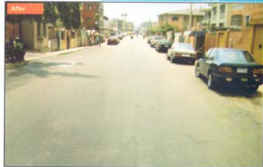
Completed 400m long Jones Street, Ebute-Metta West with double wall reinforced drainage system and concrete slab
