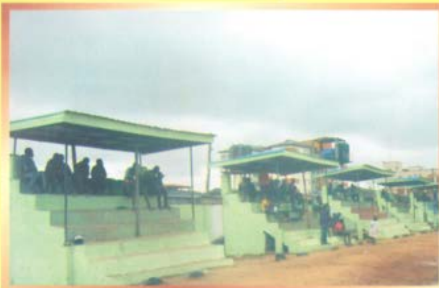
Okobaba football field pavilion after renovation
