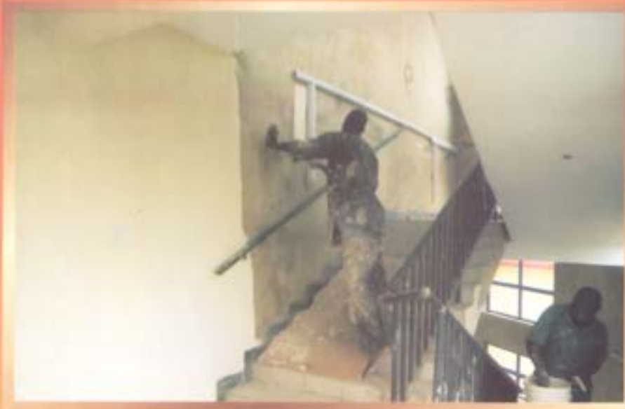
Interior painting in progress
