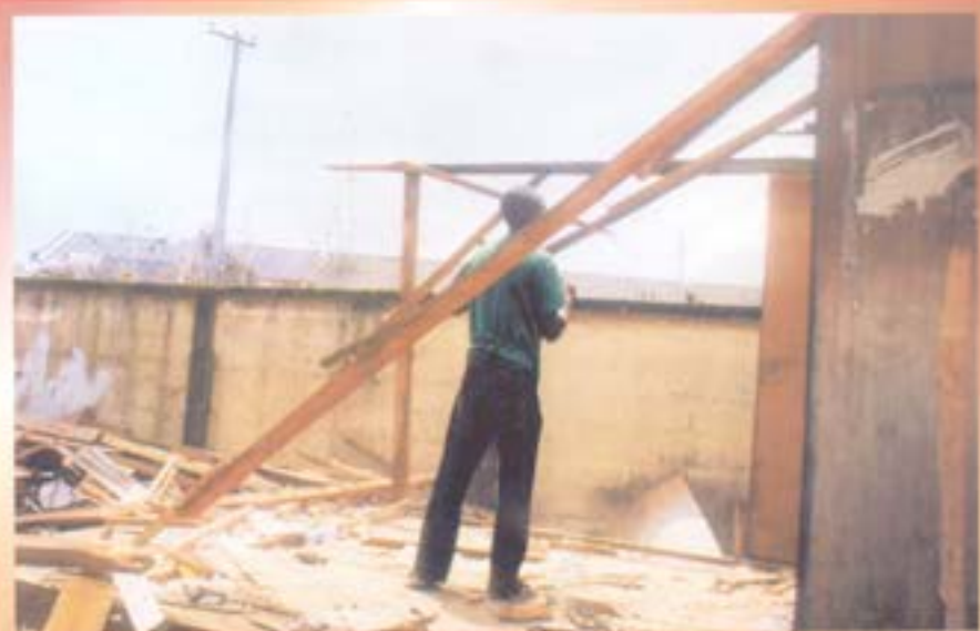
Demolition of old structures begins
