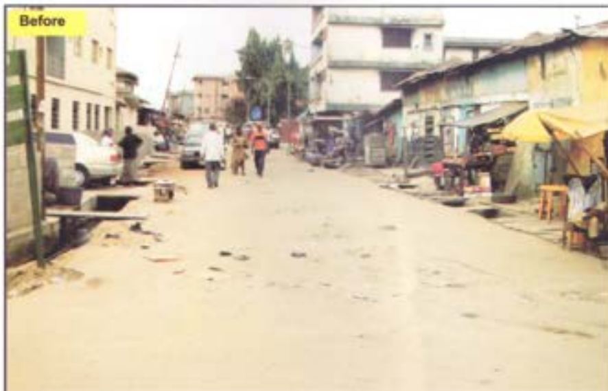
Ijero Road, Ebute-Metta West before construction
