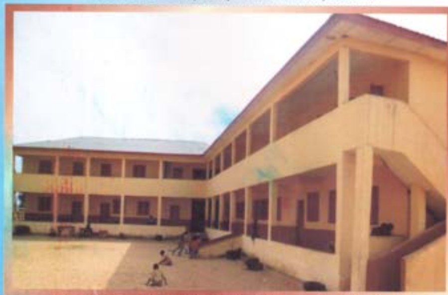
Newly completed AUD Public Primary school, Odunfa with 12 classroom, 4 toilets and 4 offices
