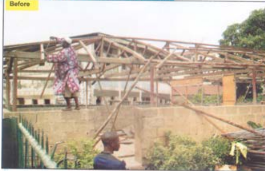
Demolition of UNA Primary School, Odunfa, Ebute-Metta East
