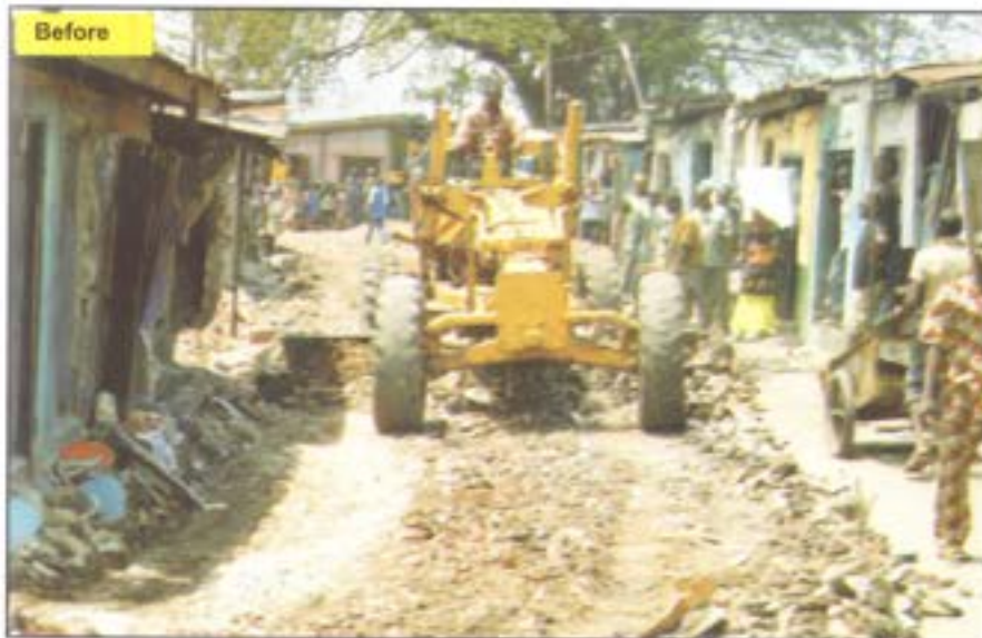
Oba Ganiyu Odesanya Road, Otto before construction
