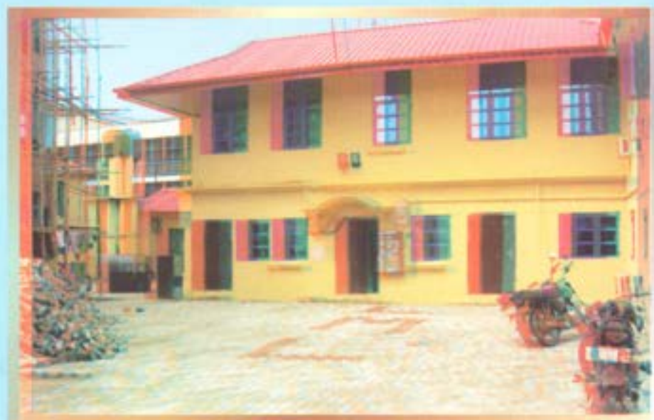
The old secretariat building with interlocking bricks after renovation
