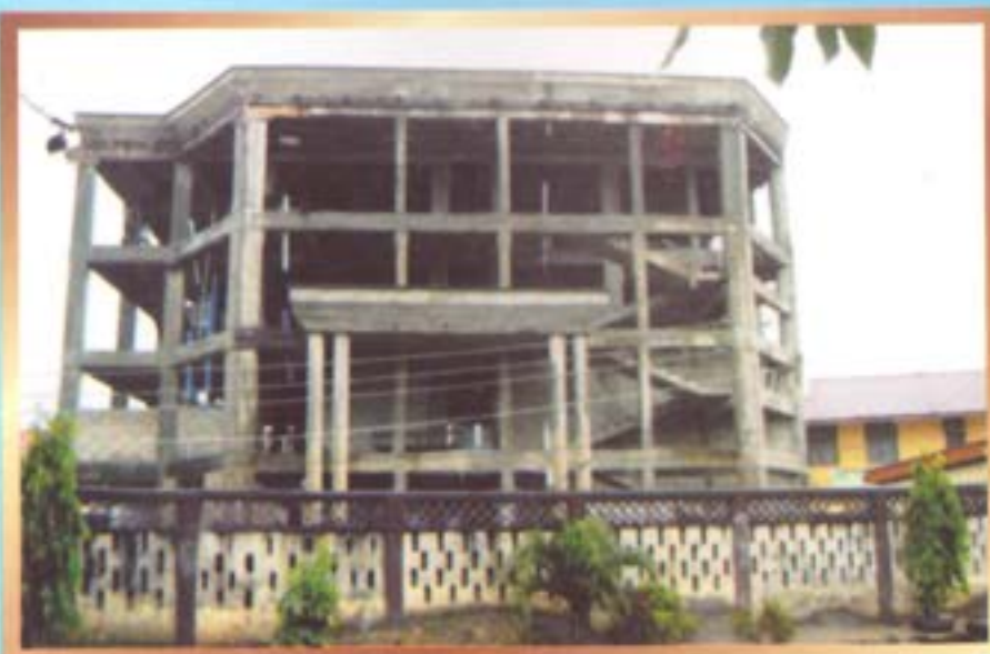
Construction work in progress (Front view)
