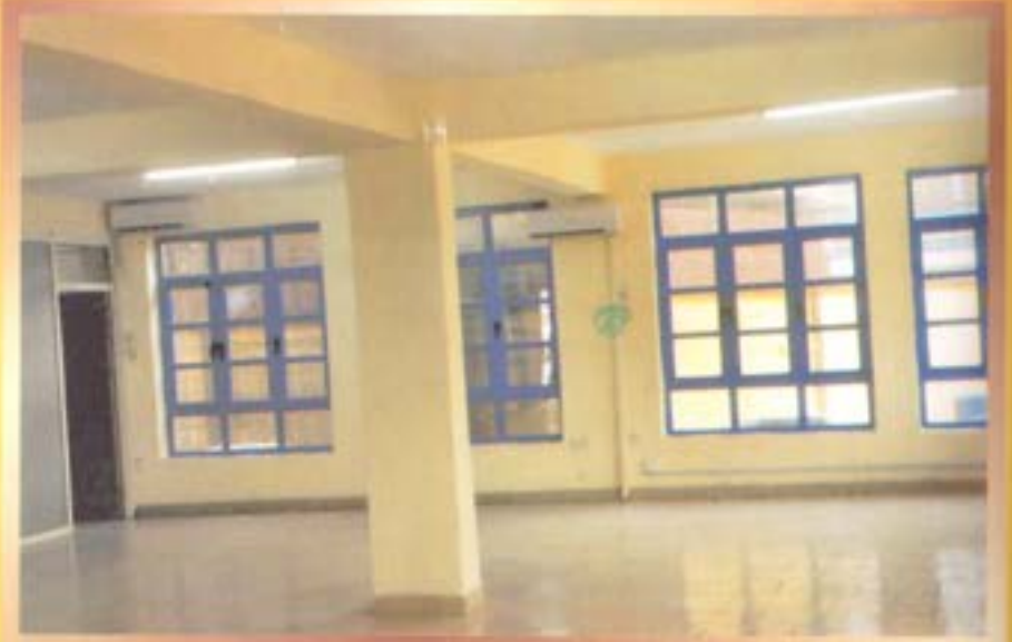
Completed floor tiling with reflective aluminum glass windows
