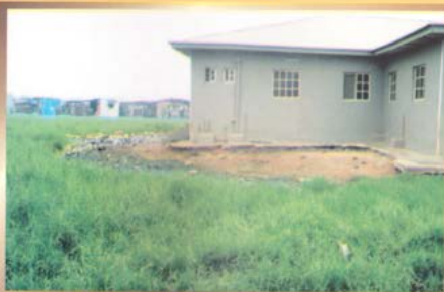
The PHC Premises before laying of Inter-Locking Stones
