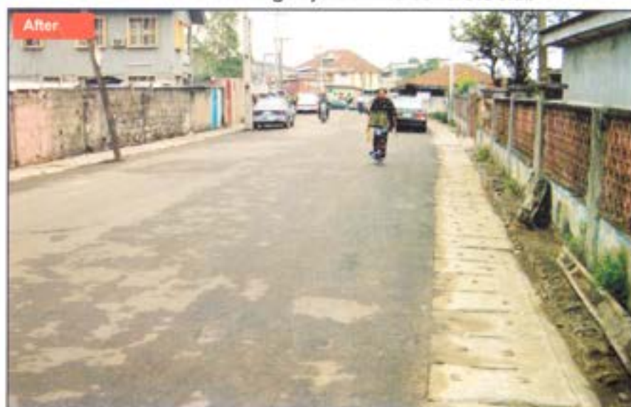
Completed 110m long New Town Road, Ebute-Metta West with double wall reinforced drainage system and concrete slab
