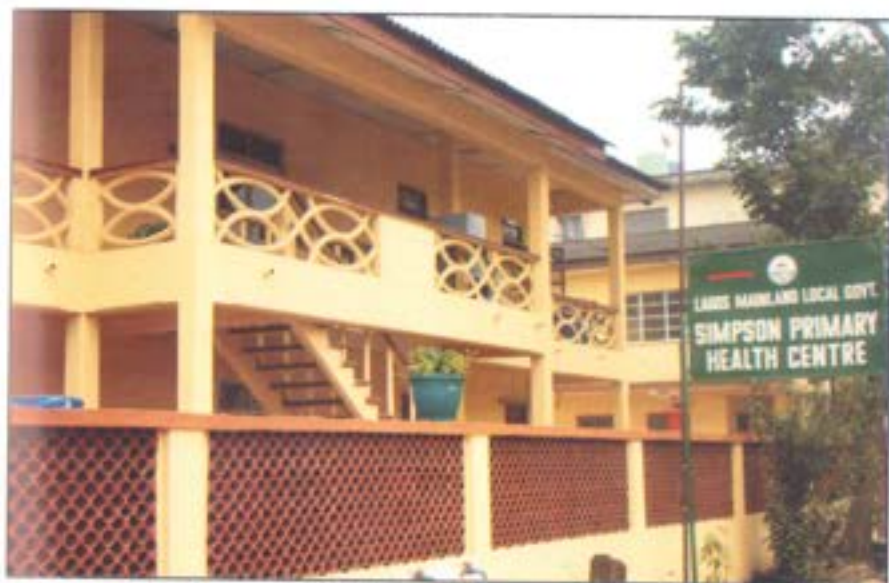
Newly renovated Simpson Primary Health Centre, equipped and upgraded for 24 hours' service
