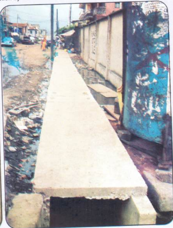
After Construction of 860m drainage system with double wall reinforced concrete and a concrete covered slab
