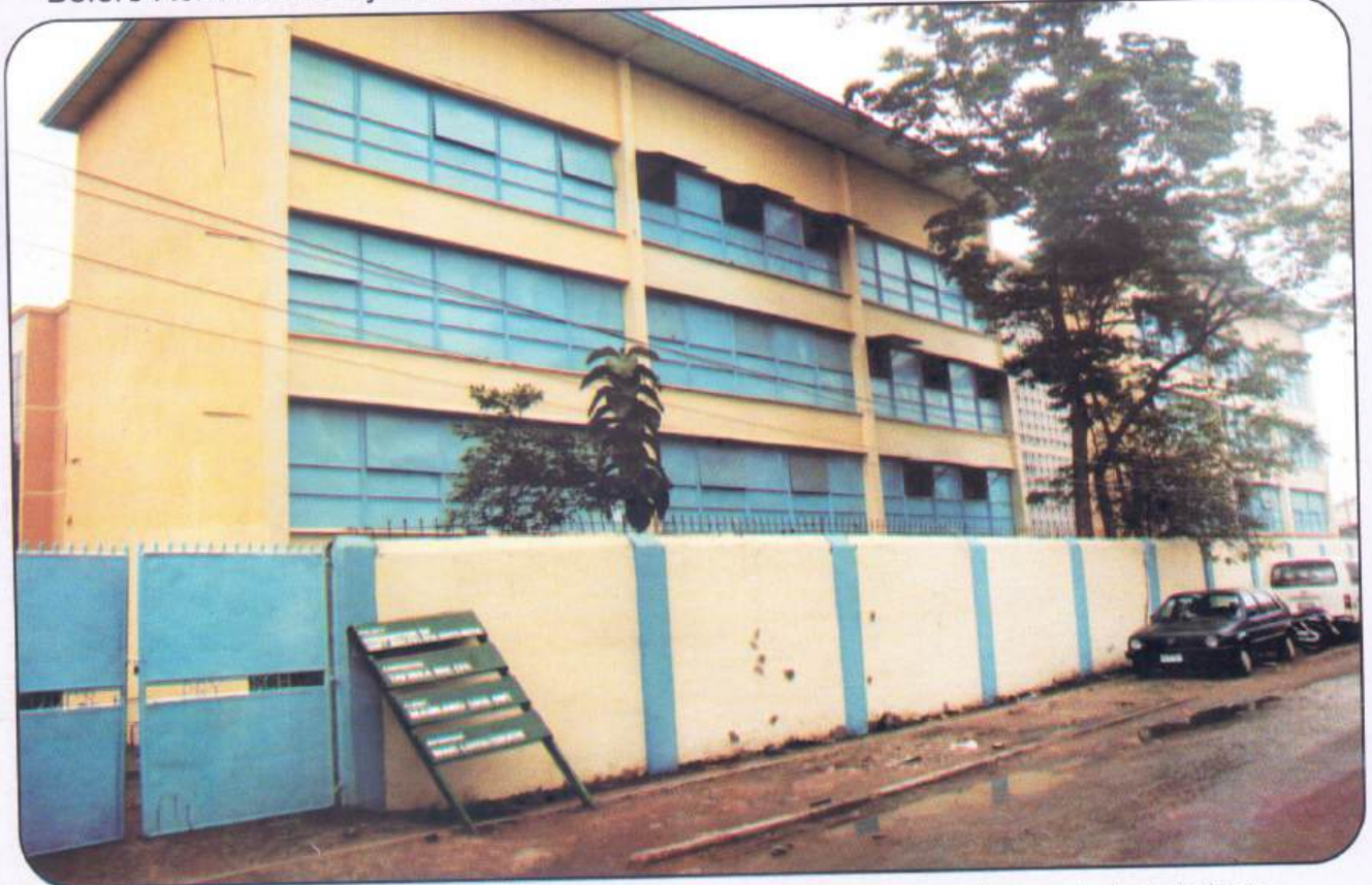
Complete Renovations - Replacement of the entire roofing system, replacement of all windows and doors, repair of all cracked walls both within and outside and general painting of the whole school
