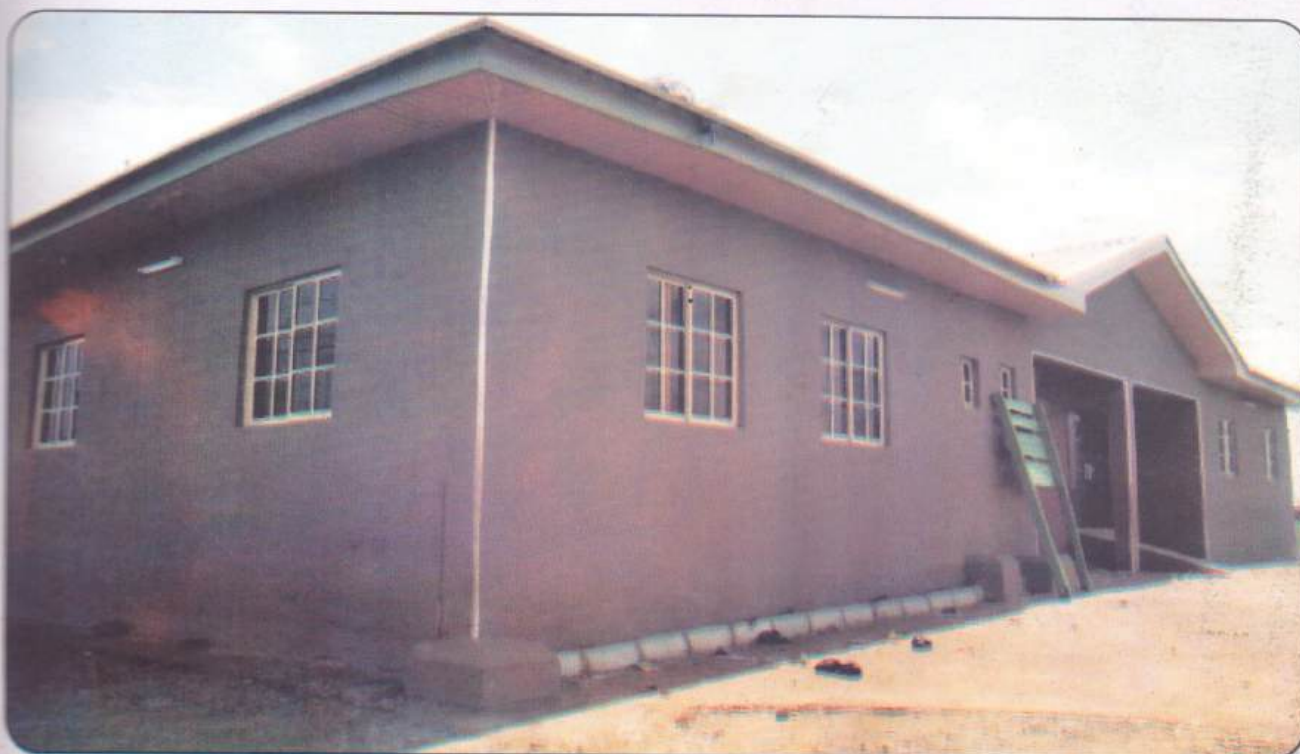
Completed with a Male & Female Ward, Pharmacy, Dispensing Room, Waiting Room, Four Doctor's Offices, Bore Hole, Bathroom and Toilet Facilities
