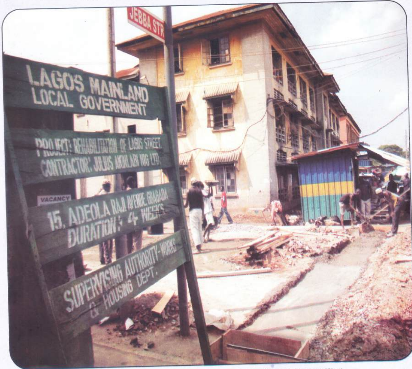
Completed Reinforced Concrete Culvert along Jebba Street Ebute-Metta West
