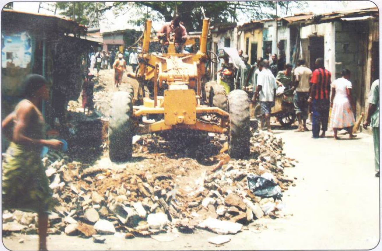
During Scarification by Lagos Mainland Local Government
