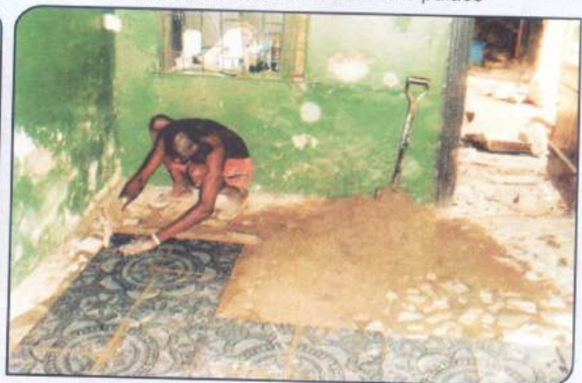
On going renovations inside the palace
