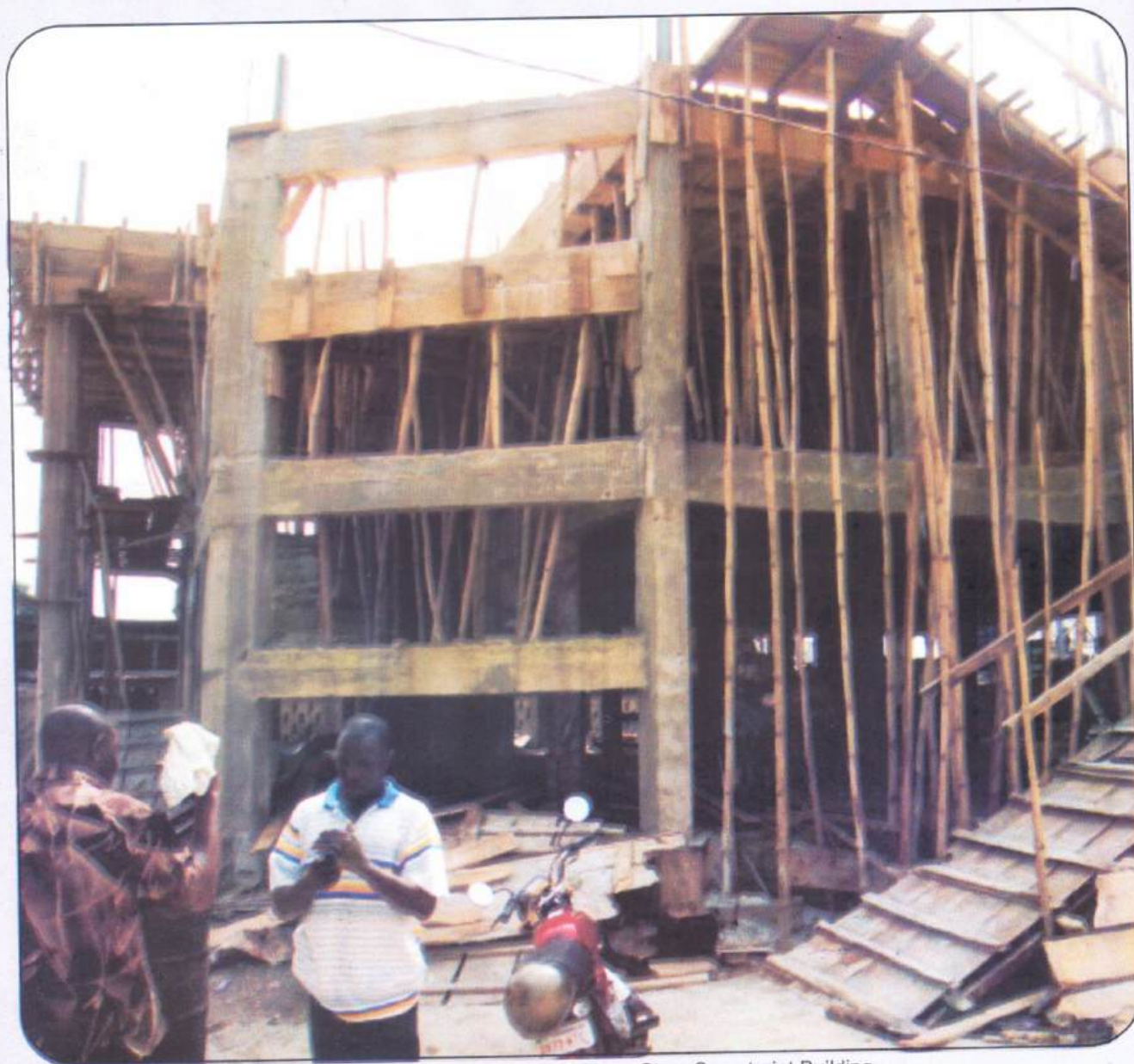
On Going Construction of New Three Story Secretariat Building
