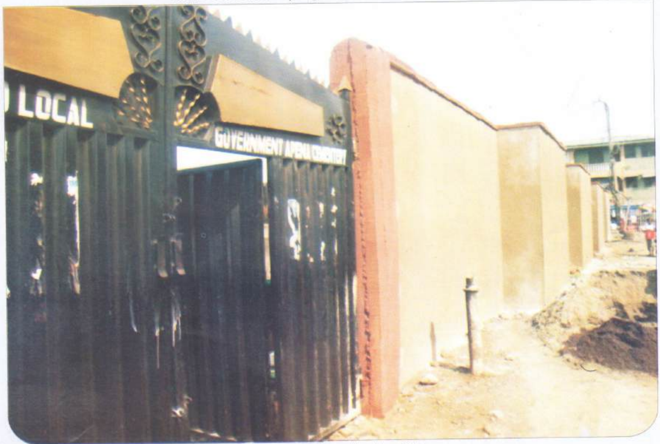
After Construction with a New Gate
