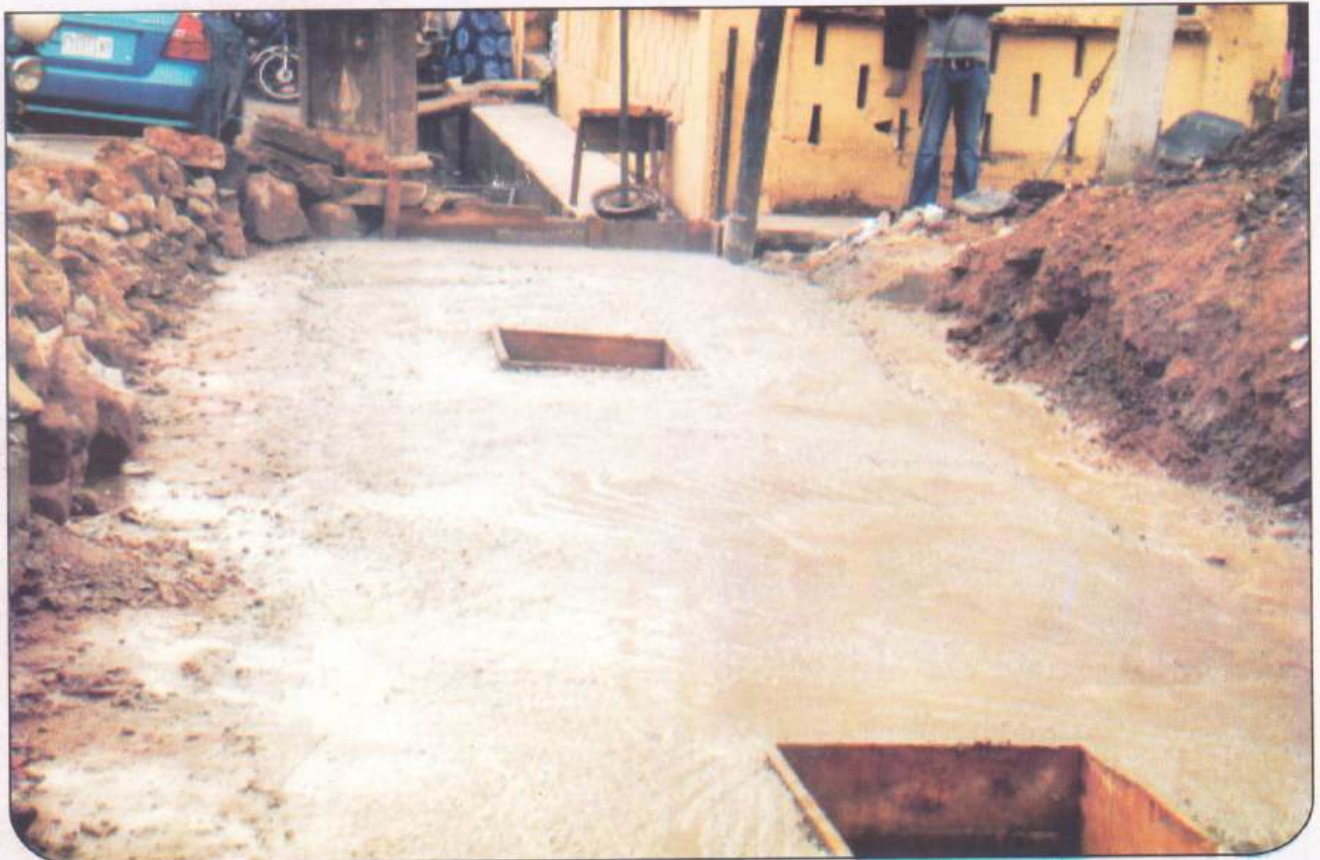
Newly Constructed Reinforced Concrete Culvert to improve the flow of water thereby eliminating flood situations
