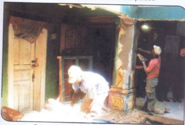
On going renovations inside the palace
