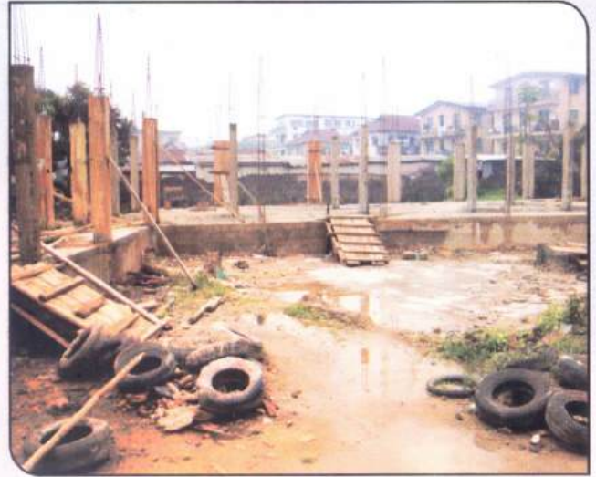
Completed Raft foundation for the new one embarked by LMLG under the leadership of Hon. Adekanye (LADO)
