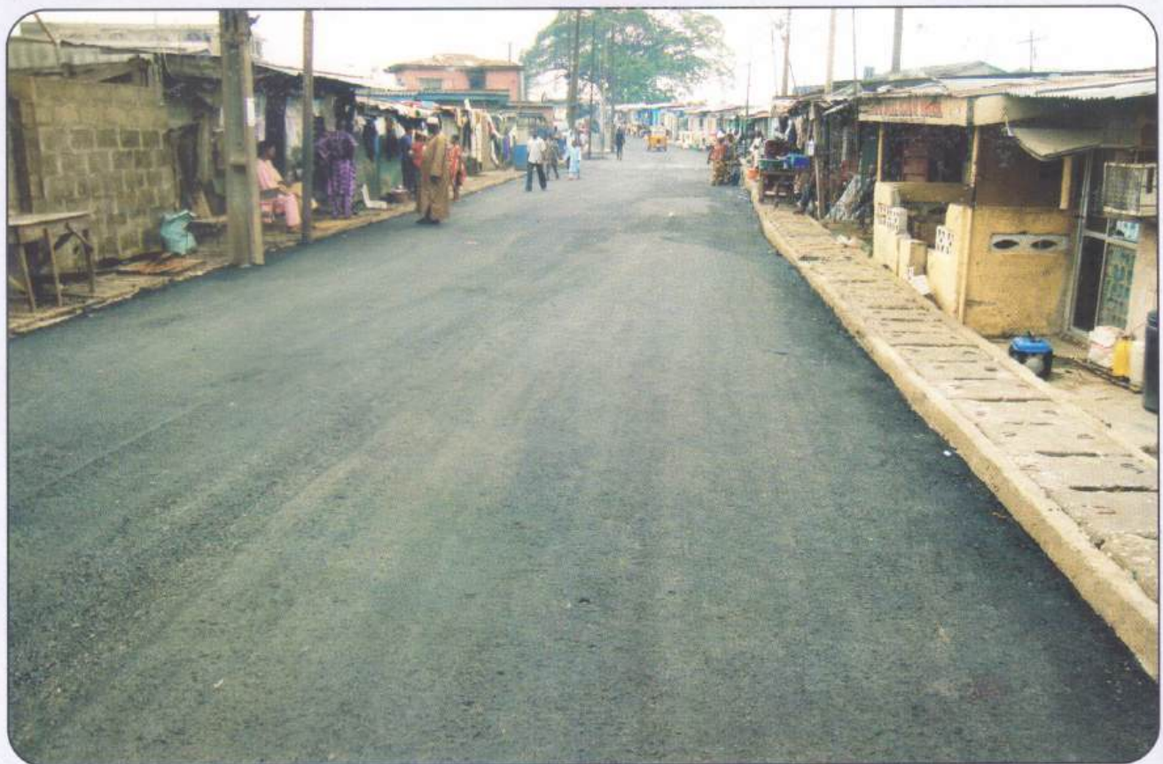
After Construction of 695m Oba Ganiyu Odesanya Road with double wall reinforced concrete drainage system and a concrete covered slab
