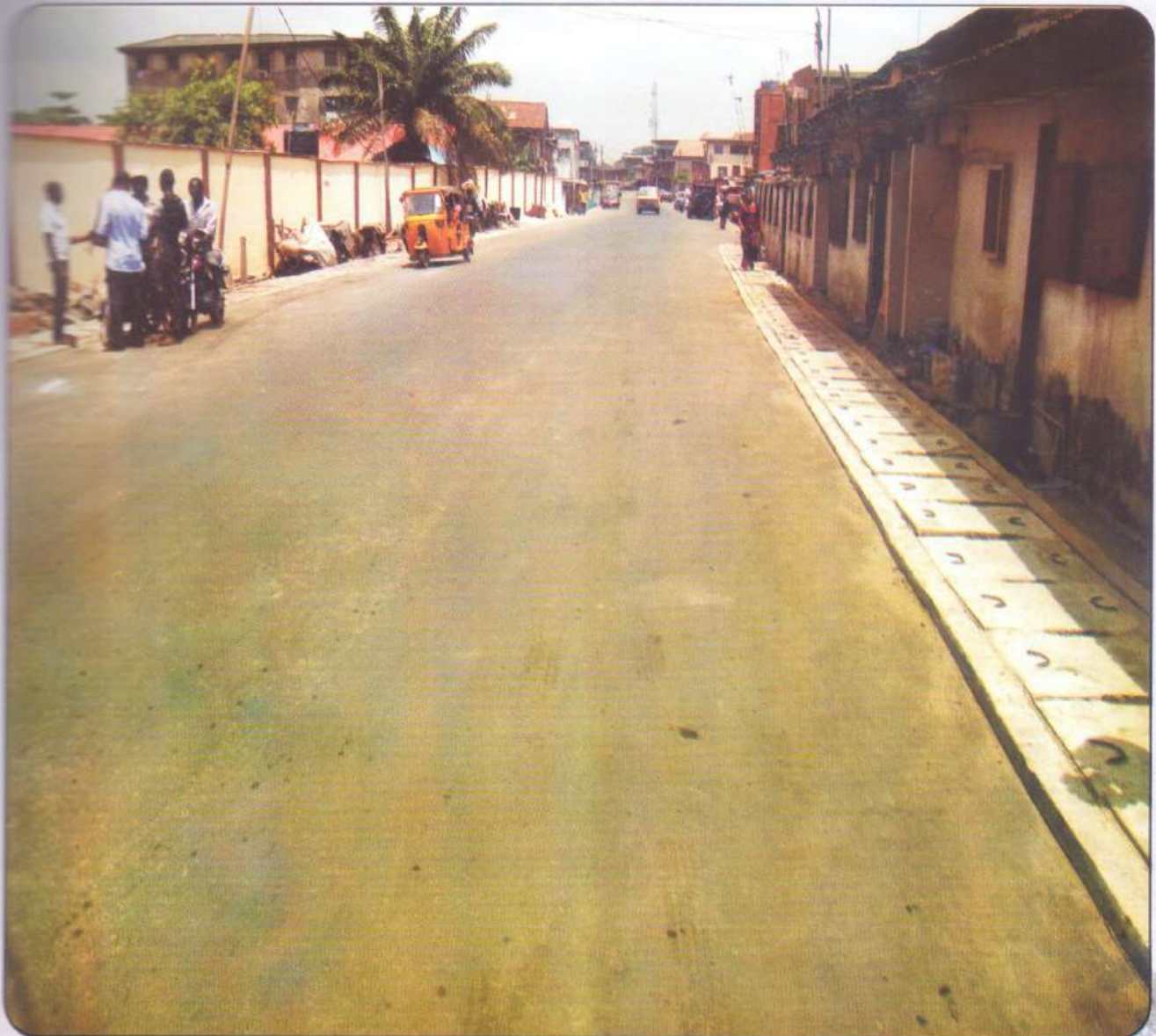
After Construction of 900m Park Road with double wall reinforced concrete drainage system and a concrete covered slab
