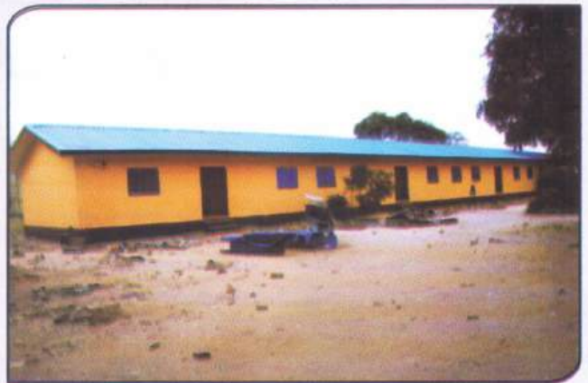
St. Paul's Catholic Primary School Hall
