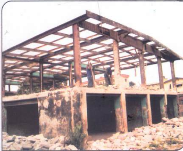
Demolition of the certified structurally defective school building at A.U.D. Primary School Odunfa
