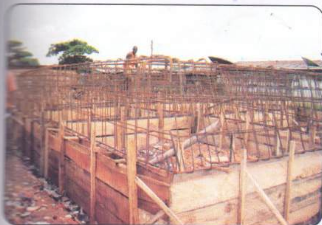
Construction of a Raft Foundation
