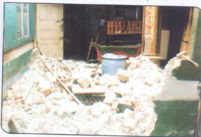
On going renovations inside the palace
