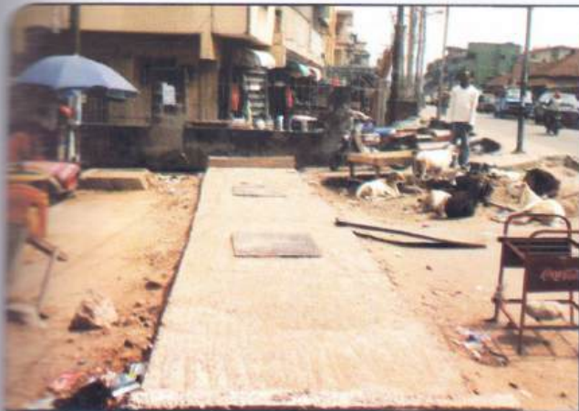
Reinforced Concrete Culvert Construction along Lagos Street by Bornu Way Ebute-Metta East
