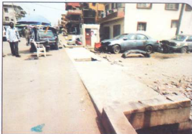
Reinforced Concrete Culvert Construction along Lagos Street by Osholake Street Ebute-Metta East
