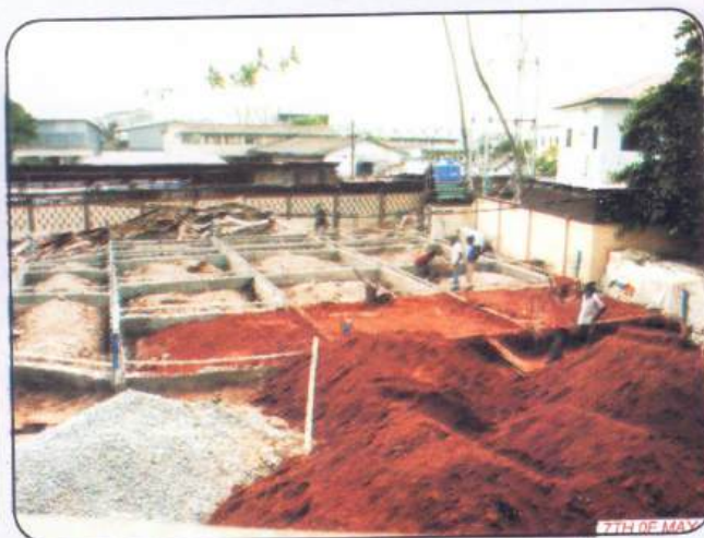
Raft Foundation in Progress
