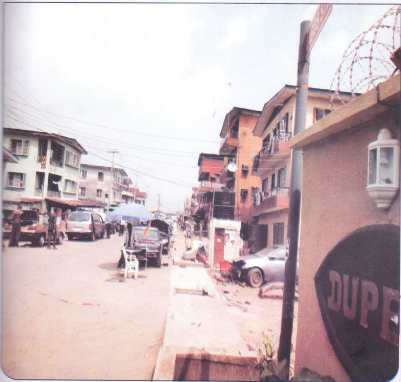
Reinforced Concrete Culvert Construction along Lagos Street Odunfa Street Ebute-Metta East
