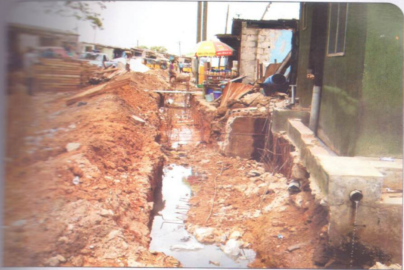
During Construction by Lagos Mainland Local Government
