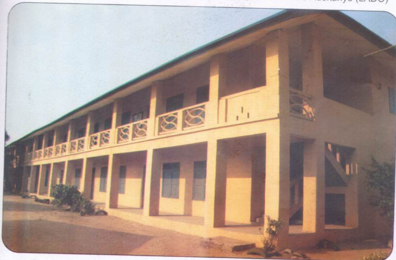
Complete Renovations - Replacement of the entire roofing system, replacement of all windows and doors, repair of all cracked walls both within and outside and general painting of the whole school
