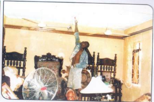
On going renovations inside the palace
