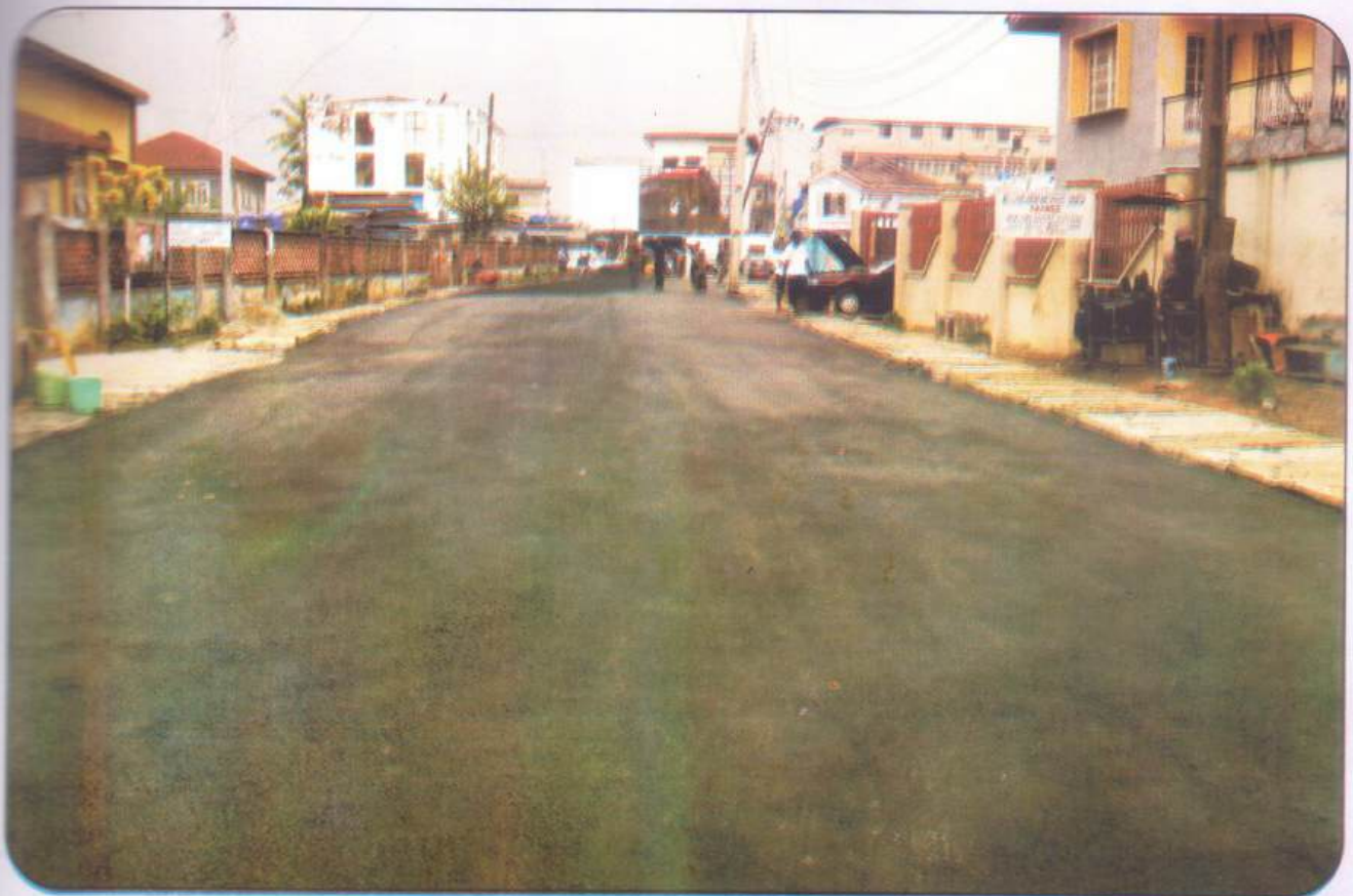
After Construction of 110m New Town Road with double wall reinforced concrete drainage system and a concrete covered slab
