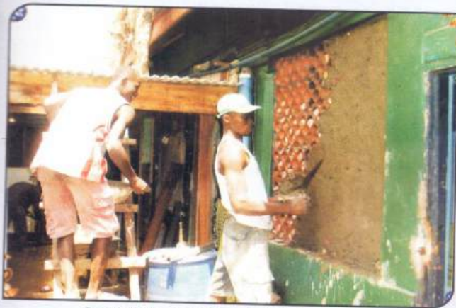
On going renovations inside the palace
