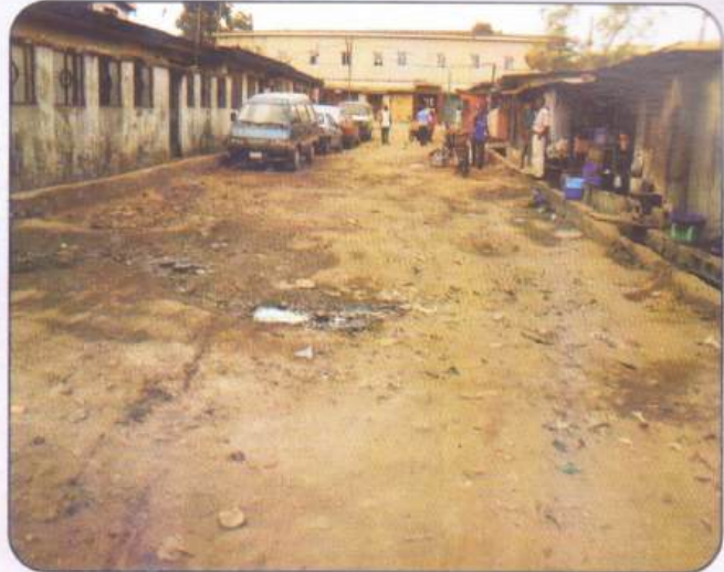
Before Construction by LMLG
