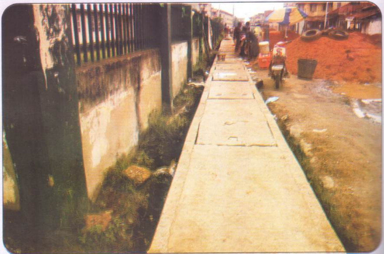
After Construction of 800m drainage system with double wall reinforced concrete and a concrete covered slab
