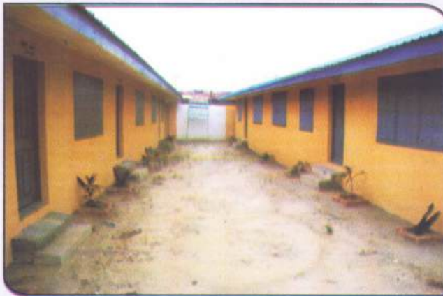
Otto Primary School (Two Blocks of Three Classroom each)
