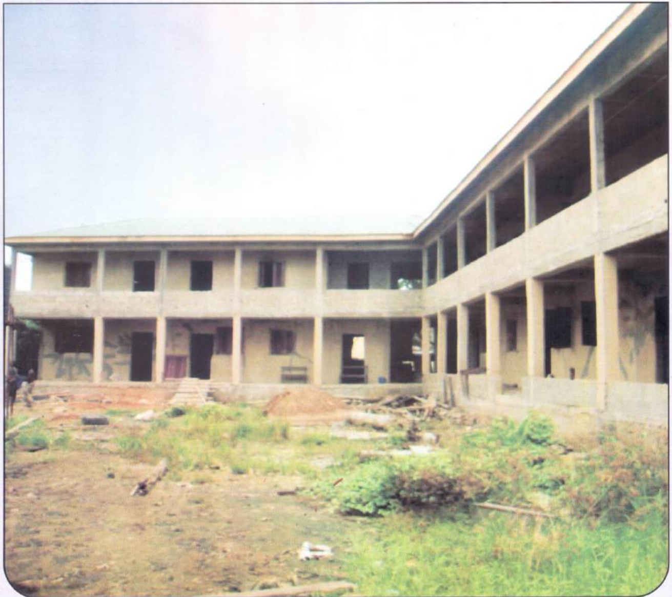
Ongoing construction of the new A.U.D. Primary School Odunfa with Ten Classrooms, Two Staff Offices and Eight Toilet facilities
