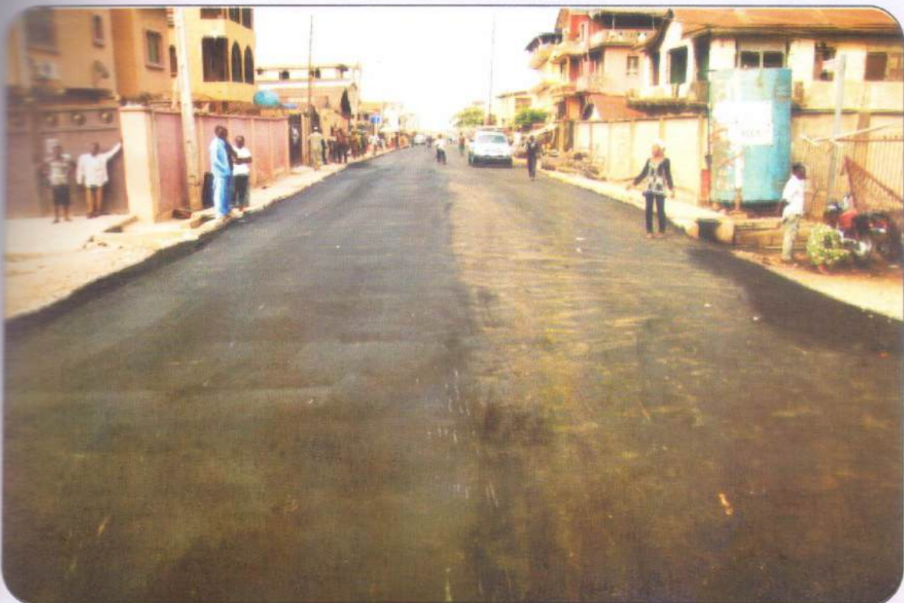
After Construction of 430m Lagos Street Road with double wall reinforced concrete drainage system and a concrete covered slab
