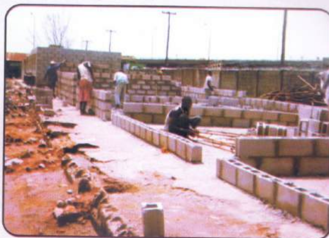
Laying a new foundation after the demolition of the existing structure
