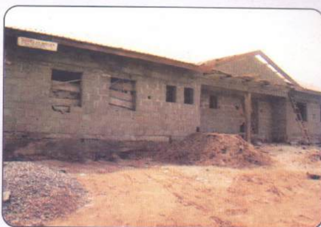
On Going Construction
